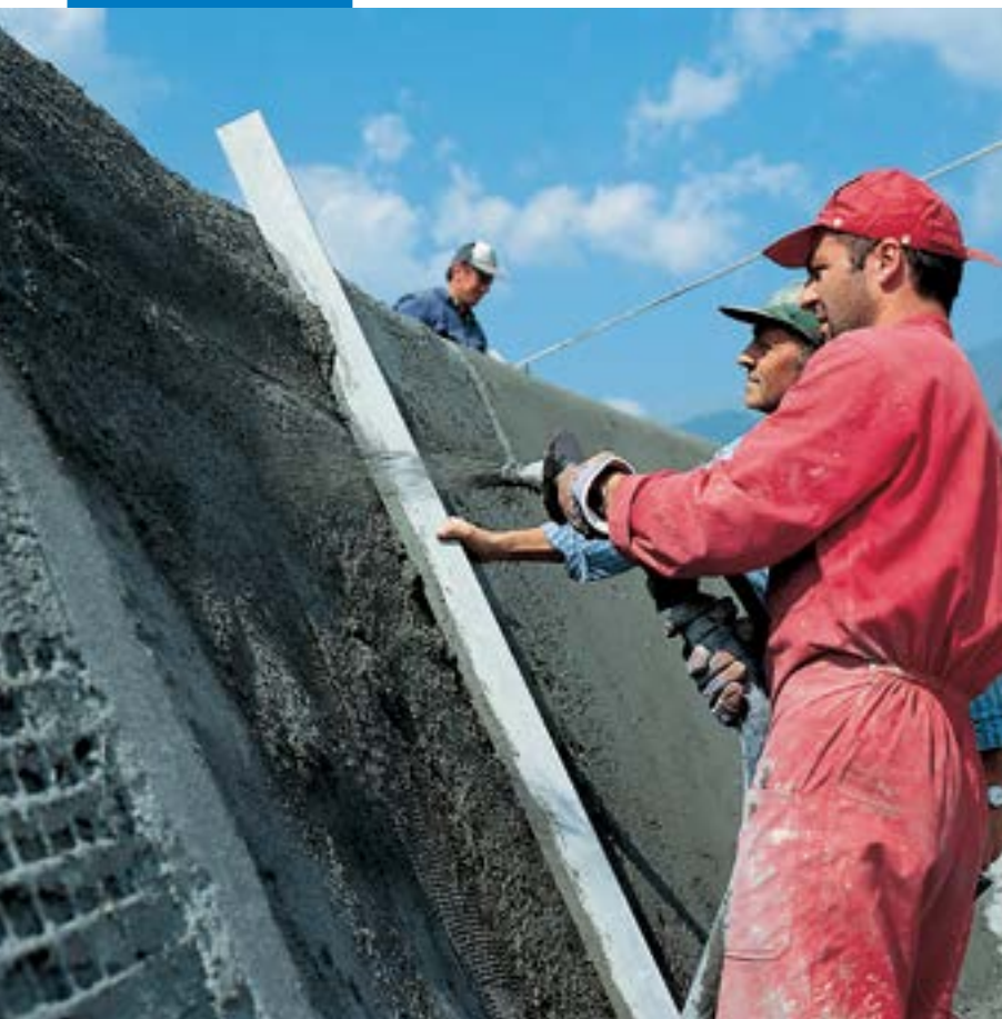
Spray application of Mapegrout T40
