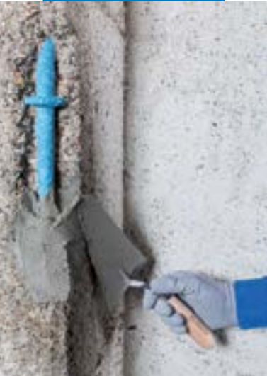
Applying Planitop Smooth & Repair R4 ZA with a trowel
