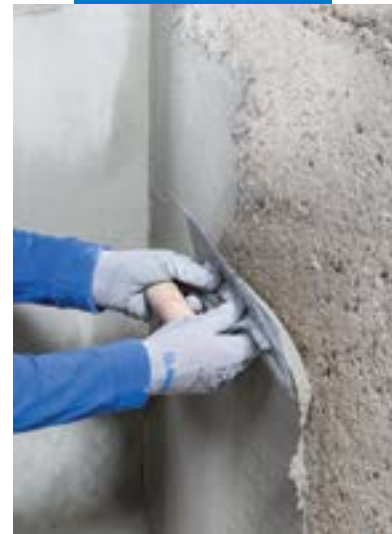
Applying Planitop Smooth & Repair R4 ZA with a putty knife
