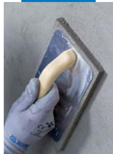
Floating the surface of Planitop Smooth & Repair R4 ZA
