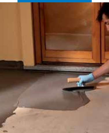
Waterproofing of terraces by trowel
