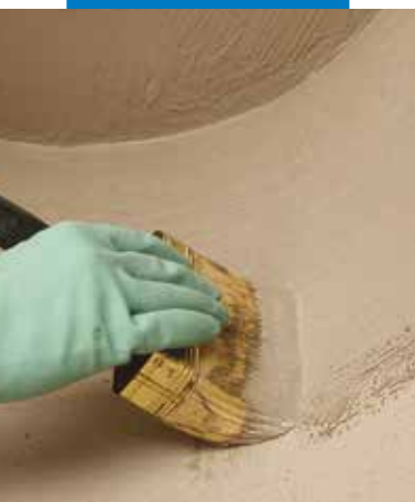
Waterproofing of details by brush
