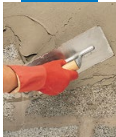
Application of Planiseal 88 by trowel
